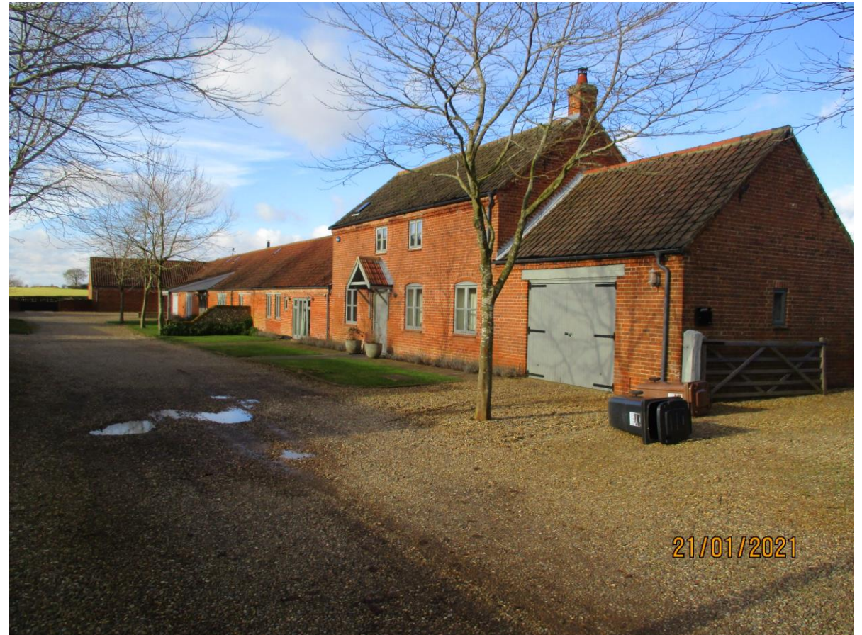
Adjacent converted barns to west
