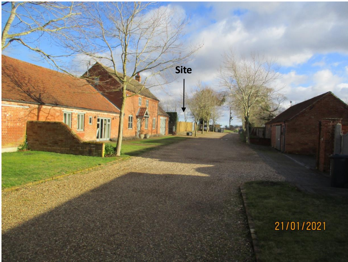
View eastwards along access
